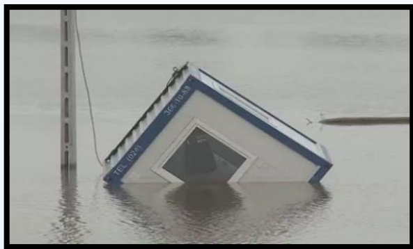
Flood affecting A1 motorway construction site. Source: GDDKiA
