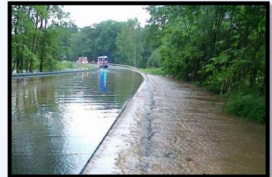
Flood in a polish local road. Source: GDDKiA
